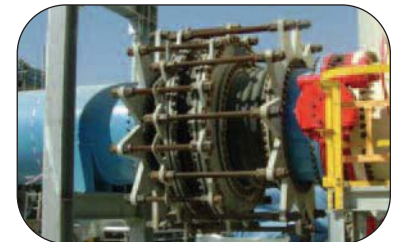
Rubber Inline Pressure Balanced Expansion Joint
