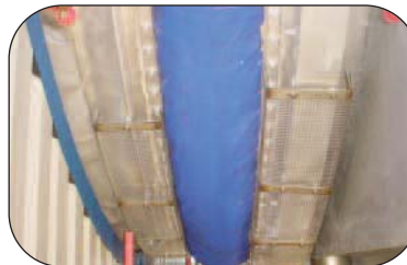
Flue Gas Corrosion Resistant Ducting Expansion Joint
