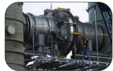
Inline Pressure Balanced Expansion Joint
